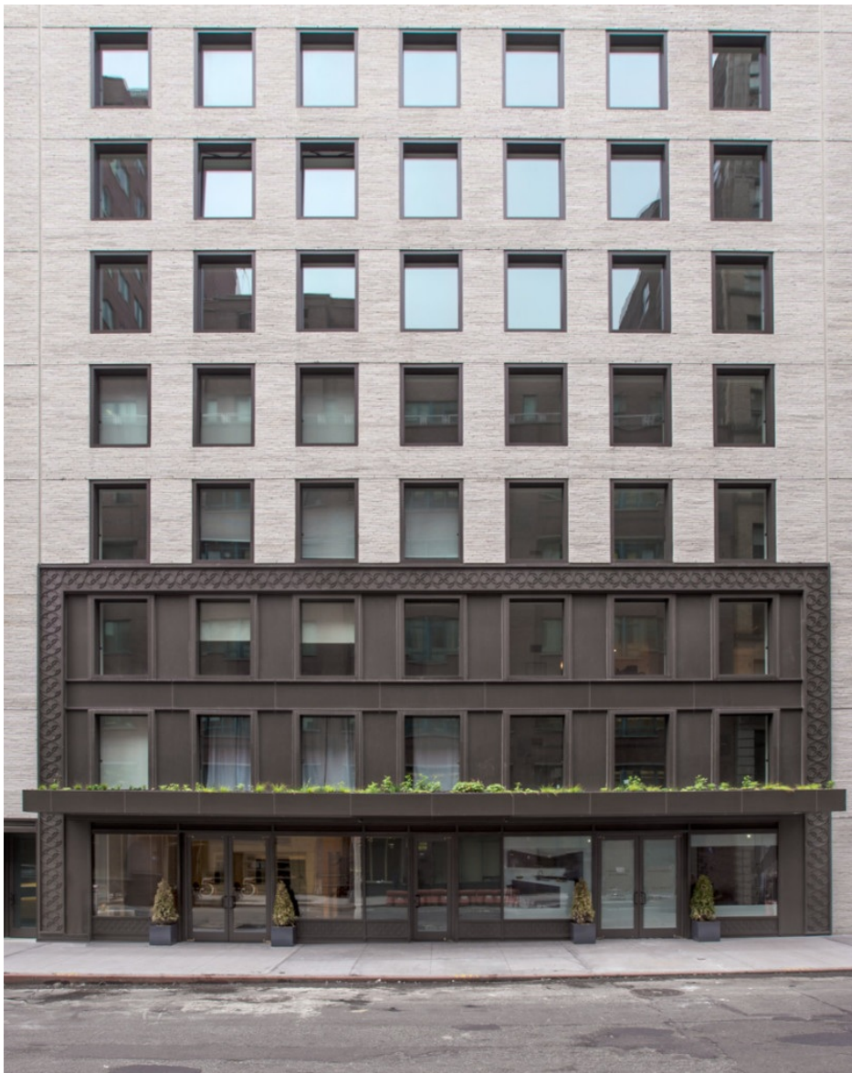
Clad in Petersen bricks, the project replaces an old office building near the Ladies' Mile Historic District in Manhattan.
