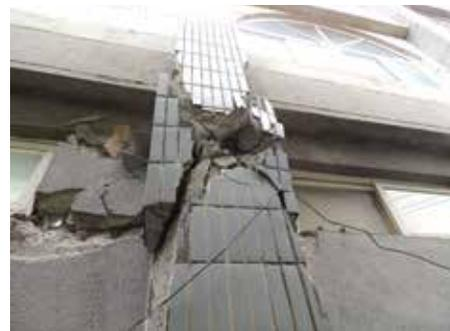
value to politicians and the general public. The need for special inspection requirements in Taiwan was highlighted in some of the failures observed, such as inconsistently spaced rebar ties and embedded architectural items in columns. Often codes and practices are developed in parallel, with each country focusing on its concerns and needs. In an increasingly global society, we need to learn from our neighbors.
