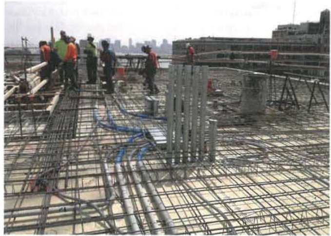
Fig. 4: By the end of day two of a 2-day construction cycle, the first portion of the subsequent slab section is ready for the next morning's concrete placement
