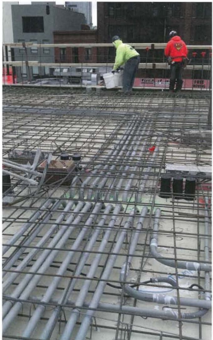
Fig. 5: Close coordination was required to avoid conflicts between the electrical conduit and reinforcing bars
