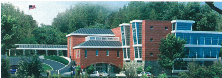
A new 45,000-sq.-ft. library facility in Ossining, N.Y., will have several green construction features, including a geothermal cooling and heating system, drought-resistant landscaping, and debris recycling.
