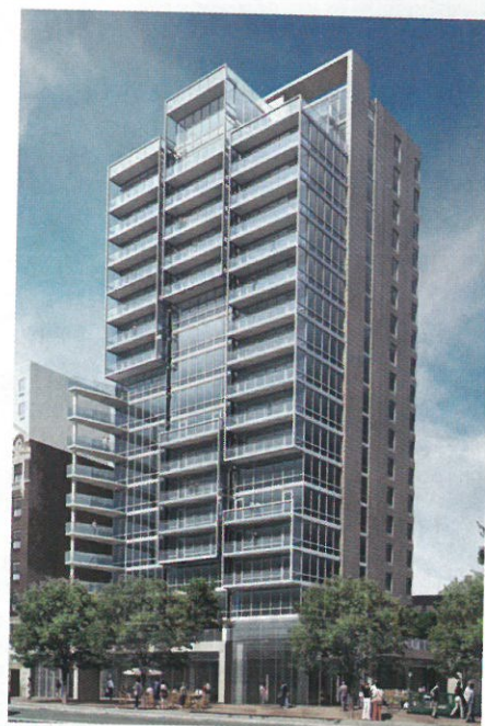
A new 47-unit, 19-story condominium building is rising on Central Park North in Manhattan.
