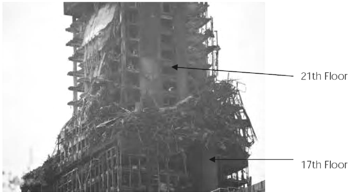
Illustration 10: Collapse Extension
