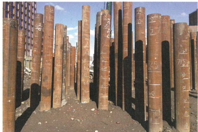
Fig. 2: Pile cluster for the core foundation walls. Over 1000 piles were required to support building columns and shear walls. The piles are tied together by a foundation slab
