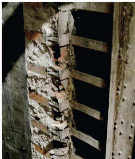
Figure 6. Existing shaft reinforcement.
