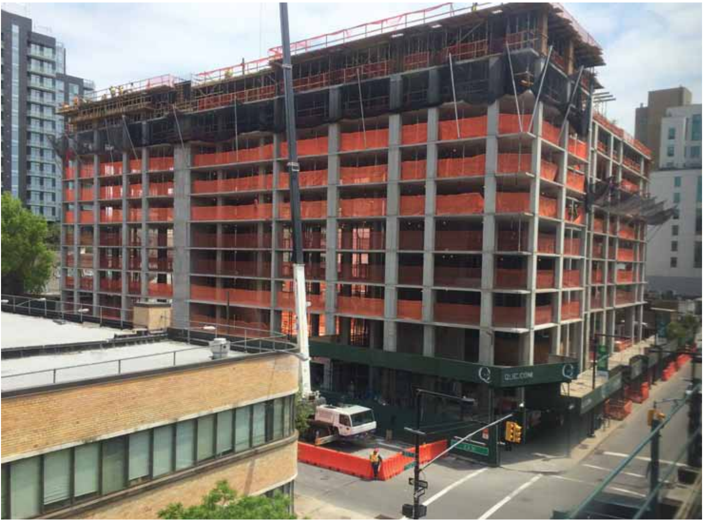
Figure 4. Flat plate concrete construction at QLIC.
