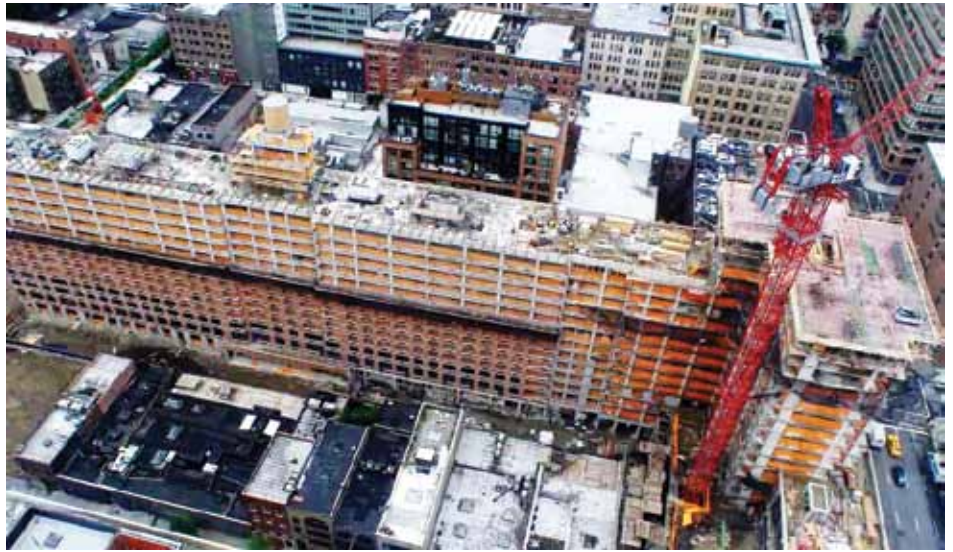
Figure 6. Avalon West Chelsea. Tower (at right) is on a 2-day cycle, with staging on mid-rise roof deck.
