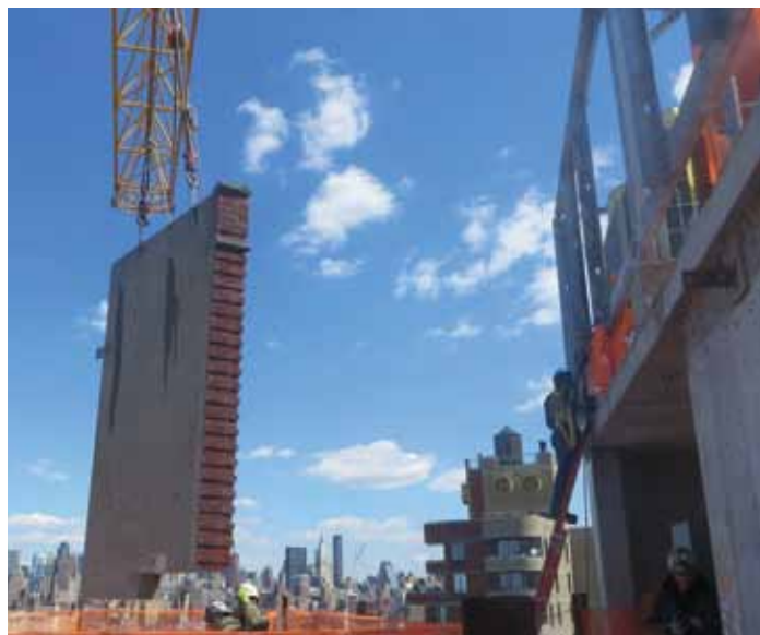
Figure 7. 13-inch precast façade panel at 150 Charles Street.
